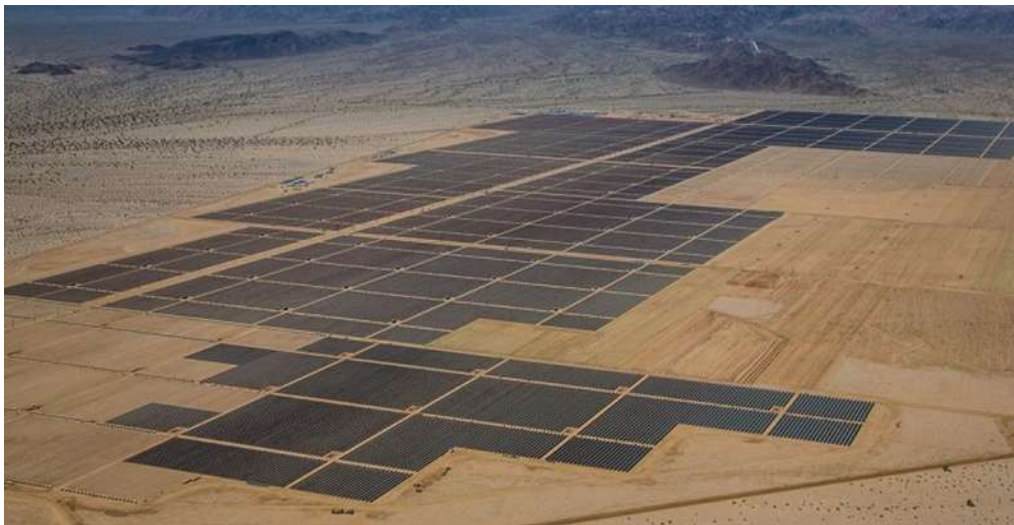
Figure 1.2: Desert Sunlight Solar Farm, a 550 MW capacity power plant in California, USA. Estimated capital cost of this facility exceeds 800 million USD based on a capex of 1.60 USD/W. Image source: Fortune, 2016.
