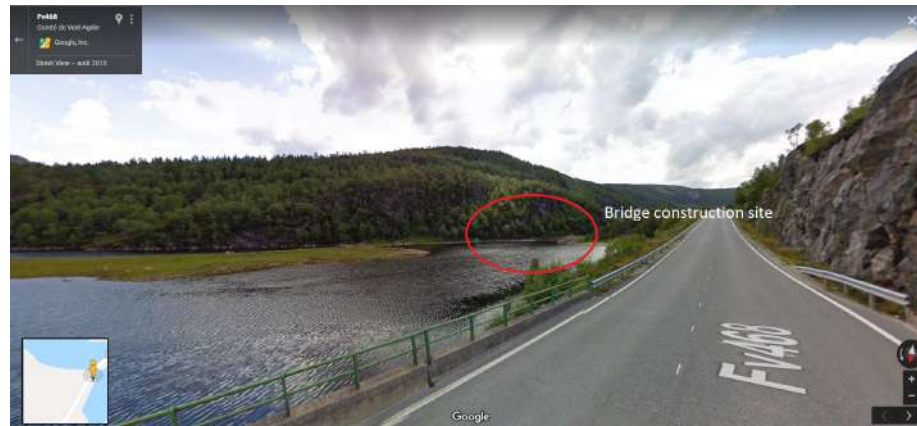
Figure 2.6: Bridge construction site
