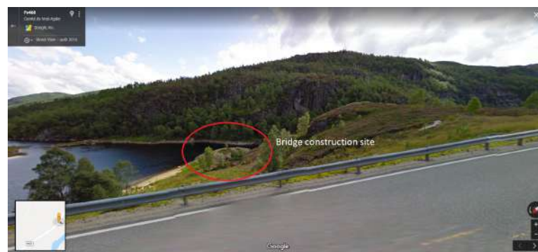
Figure 2.7: Bridge construction site
