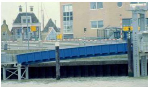
Figure 1.1: First FRP (pedestrian) bridge in Harlingen [28]
