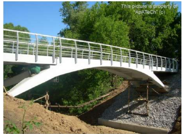
Figure 4.14: Apatech footbridge in Moscow [1]
