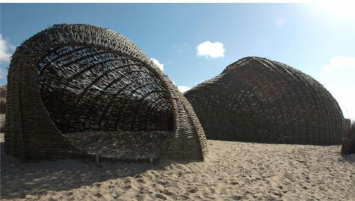
**Figure 5.5:** Large double curved domes made through weaving
