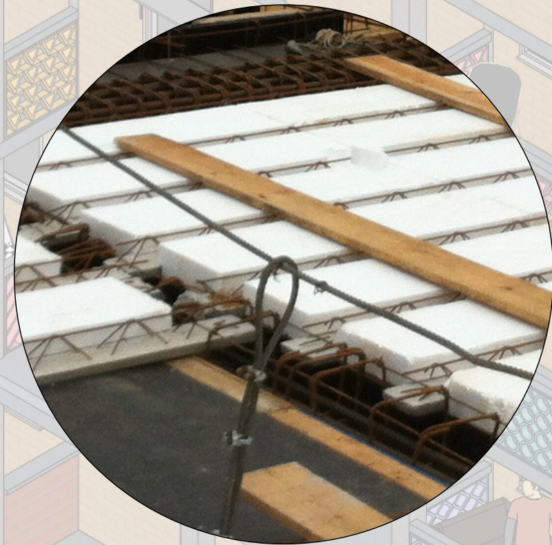
floors: recycled concrete + EPS
