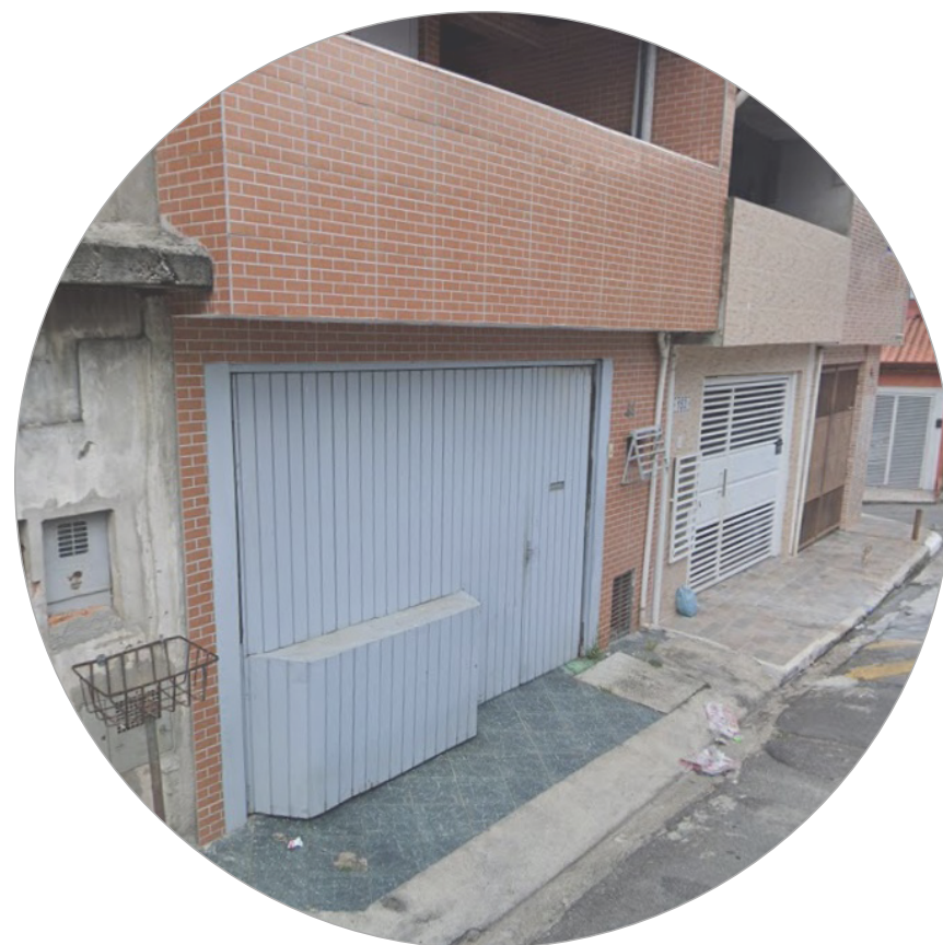
disconnection public and private on GF garages, walls, iron rasters
