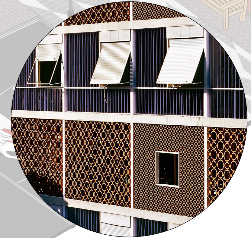
porous facades: Cobogó • cross-ventilation and shading • ceramic/concrete/fiber cement
