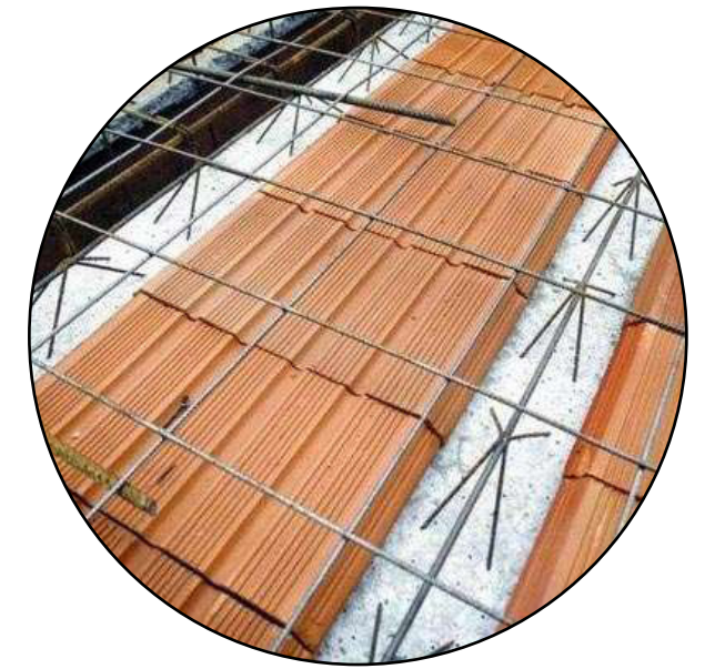
rebars before pouring concrete
