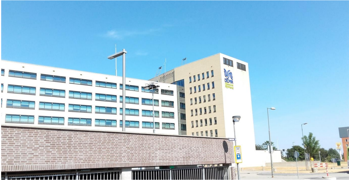
Figure 22 Overview of the newly built DCMR-office which is located at the north of the train station.
