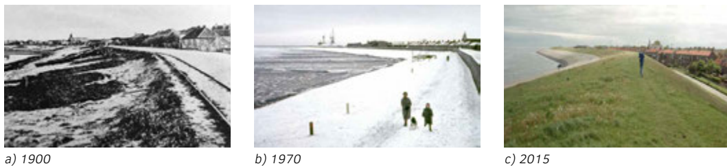
FIG. 1.3 The seawall at Den Helder in 1900 (left), 1970 (middle) and 2015 (right). Due to coastal reinforcement, the seaside setting of the fishing village was disrupted over time, cutting the town off from the sea with a 12m-high sea wall. Sources: E. de Jong (middle) and Rijkswaterstaat / Simon Warner (right).
