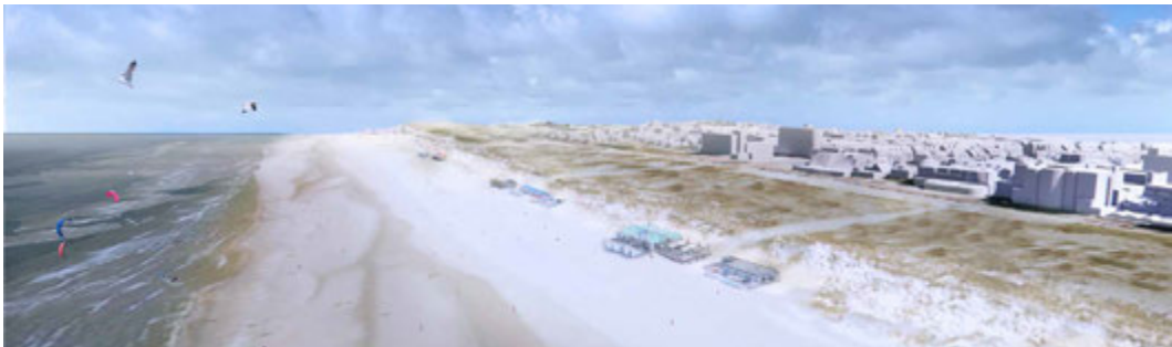
c) Noordwijk as a Sand Buffer phase 2 reinforcement, promoting BwN-based dune widening
