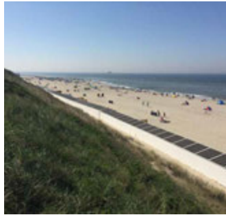
The current beach profile of Domburg, which could be sustained by the nearby mega-nourishment feeding the shore with sediment. The current beach row housing is blocking sediment transport to the foredunes, retaining a steep coastal profile. The buildings' typology could be altered to allow for more sediment transport to pass through (e.g. wider gaps or diagonal slats).
