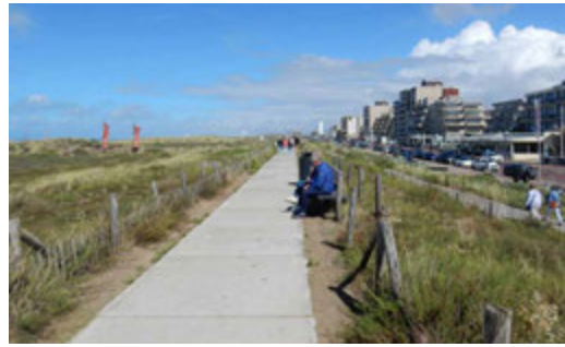
FIG. 2.10 Dike in dune reinforcement of the coastal resort in Noordwijk (right). Photo by the author.
