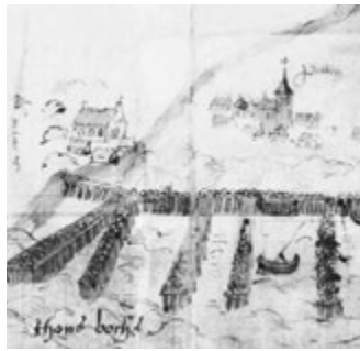
b) The village of Petten around 1552 by Jan van Scorel, with pole construction as the last sea defence.
