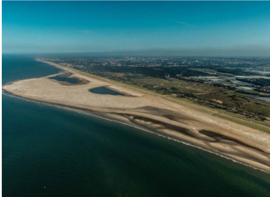
FIG. 4.46 Aerial photograph of the Sand Motor mega-nourishment just after construction in 2012, showing accretion on the south side. Source: © Rijkswaterstaat / Joop van Houdt
