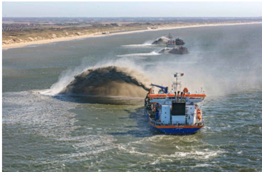
FIG. 3.6 Shoreface nourishment on the North Holland coast, Netherlands (2020). Source: © Rijkswaterstaat.
