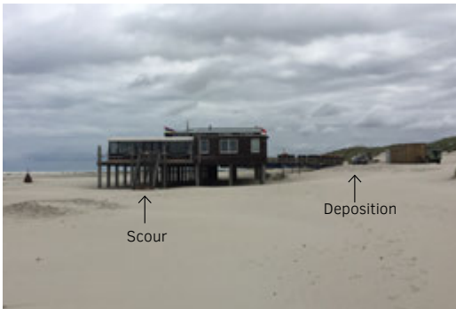
FIG. 3.26 Photograph of the year-round beach pavilion 'De Branding' at Terschelling (2018, 4 m-high poles). Visible is the scour below the pavilion resulting from local wind acceleration, as well as downwind deposition (right) in the dominant NW direction. Due to maintenance, not all deposition remains. Image by the author.
