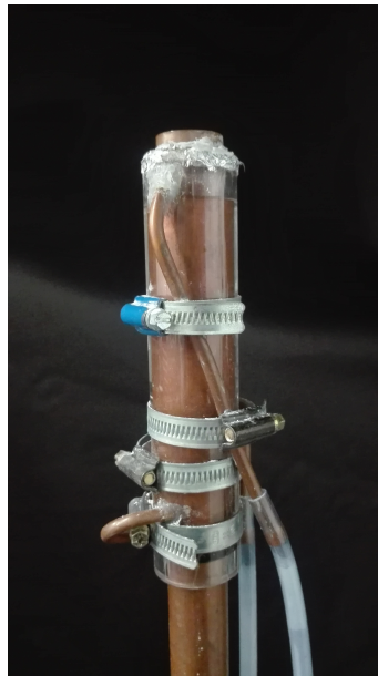
Figure 4.2: One of the cooling jackets installed on a tube burner. Tap water enters from the bottom and leaves from the top to avoid air accumulation in the device.
