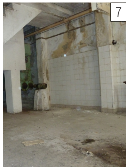
Building 16 and 16A: drainage problems at the connections between the buildings resulting in water damage on the inside of building 16, 16A and building 17.
