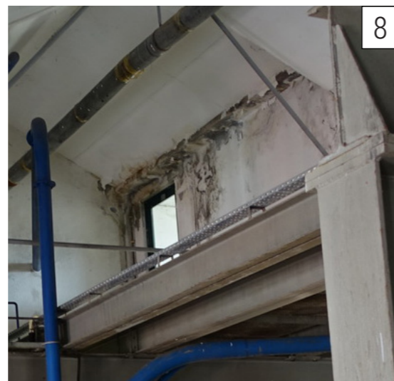
Building 18 and 19: water damage caused by leakages and badly detailed windows.
