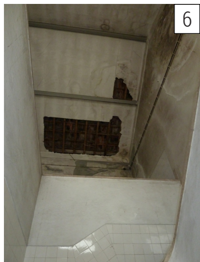
Building 16 and 16A: drainage problems at the connections between the buildings resulting in water damage on the inside of building 16, 16A and building 17.
