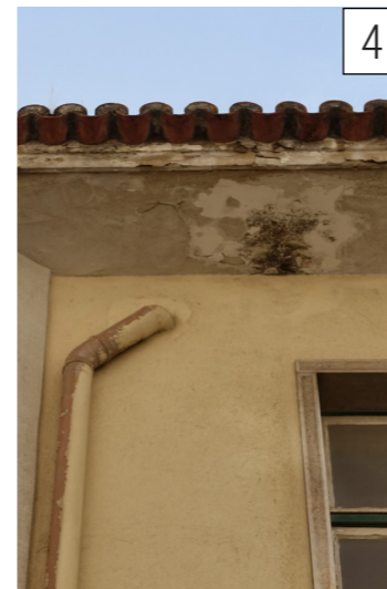
Building 16: the bakery has some drainage issues, resulting in leakages which are causing local water damage.
