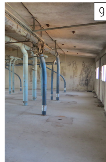
Building 18 and 19: water damage caused by leakages and badly detailed windows.
