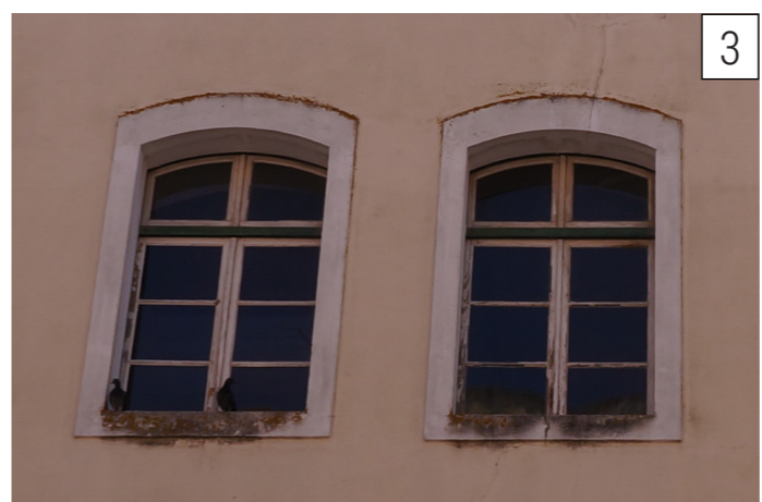
Images 1. First floor milling (photo by Hielkje Zijlstra, 04-09-2016) 2. First floor milling (photo by Hielkje Zijlstra, 04-09-2016) 3. Exterior milling first floor (photo by Jeroen van Lier, 06-09-2016)
