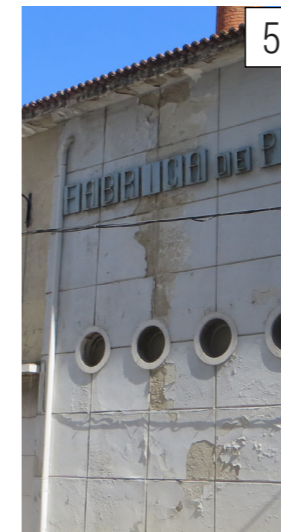
Building 16: the bakery has some drainage issues, resulting in leakages which are causing local water damage.
