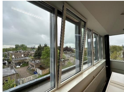
Figure 29: Tilted openable window
