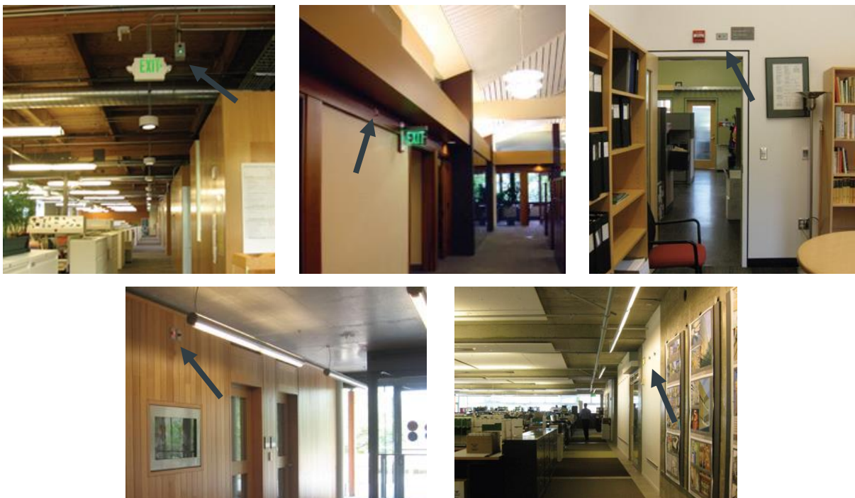
Figure 2: Encountered signalling devices by Ackerly and Brager which are not placed effectively and are easily overlooked when working. The shown signalling devices are placed far from the window and/or on the opposite side of the window (Ackerly & Brager, 2011)
