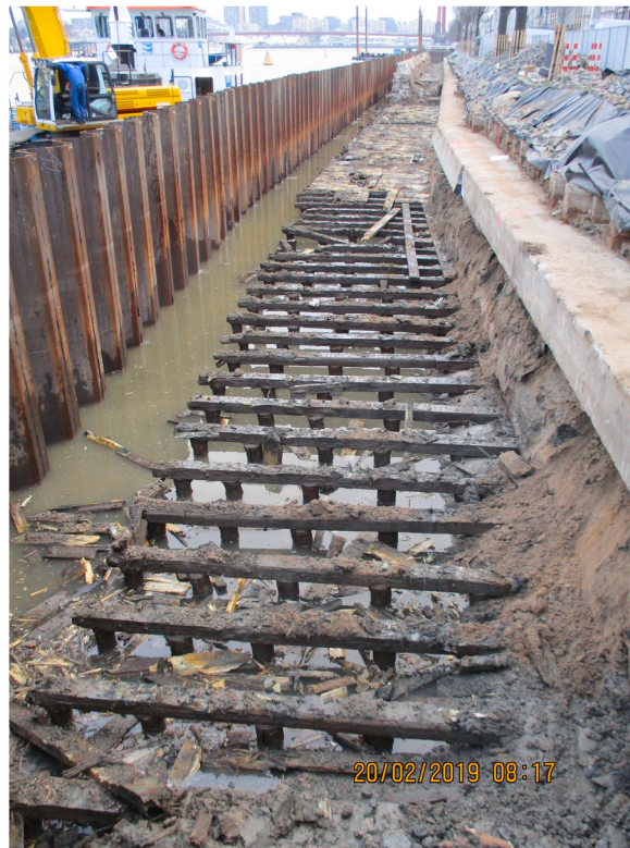
Fig. 2. Excavated historical quay wall, 'Maaskade' in Rotterdam. Photograph: Julianus, Eric. "Exposed timber pile foundation of the Maaskade". 2019. Havenbedrijf Rotterdam.
