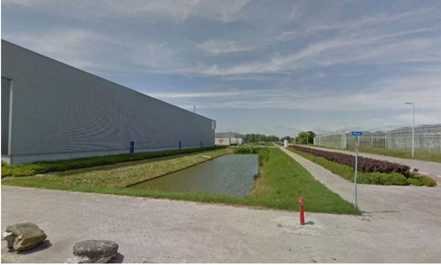
Fig. 7.9 Street view of current situation at design location, Kulkweg Hoek van Holland (Van den Brink 2021)
