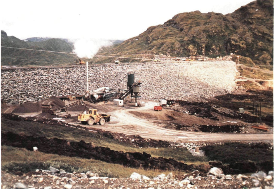
Fig. 4.2 The batch plant erected close to the downstream toe of Riskallvatn Dam
