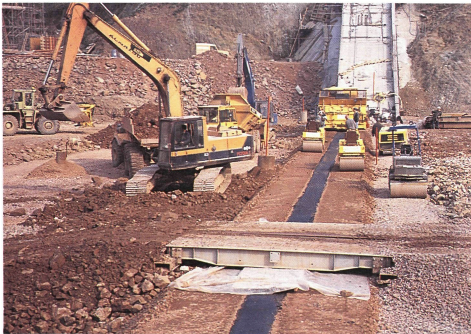
Fig. 4.8 Light steel bridge across the core
