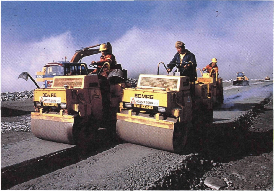
Fig. 4.4 Simultaneous compaction of core and filters
