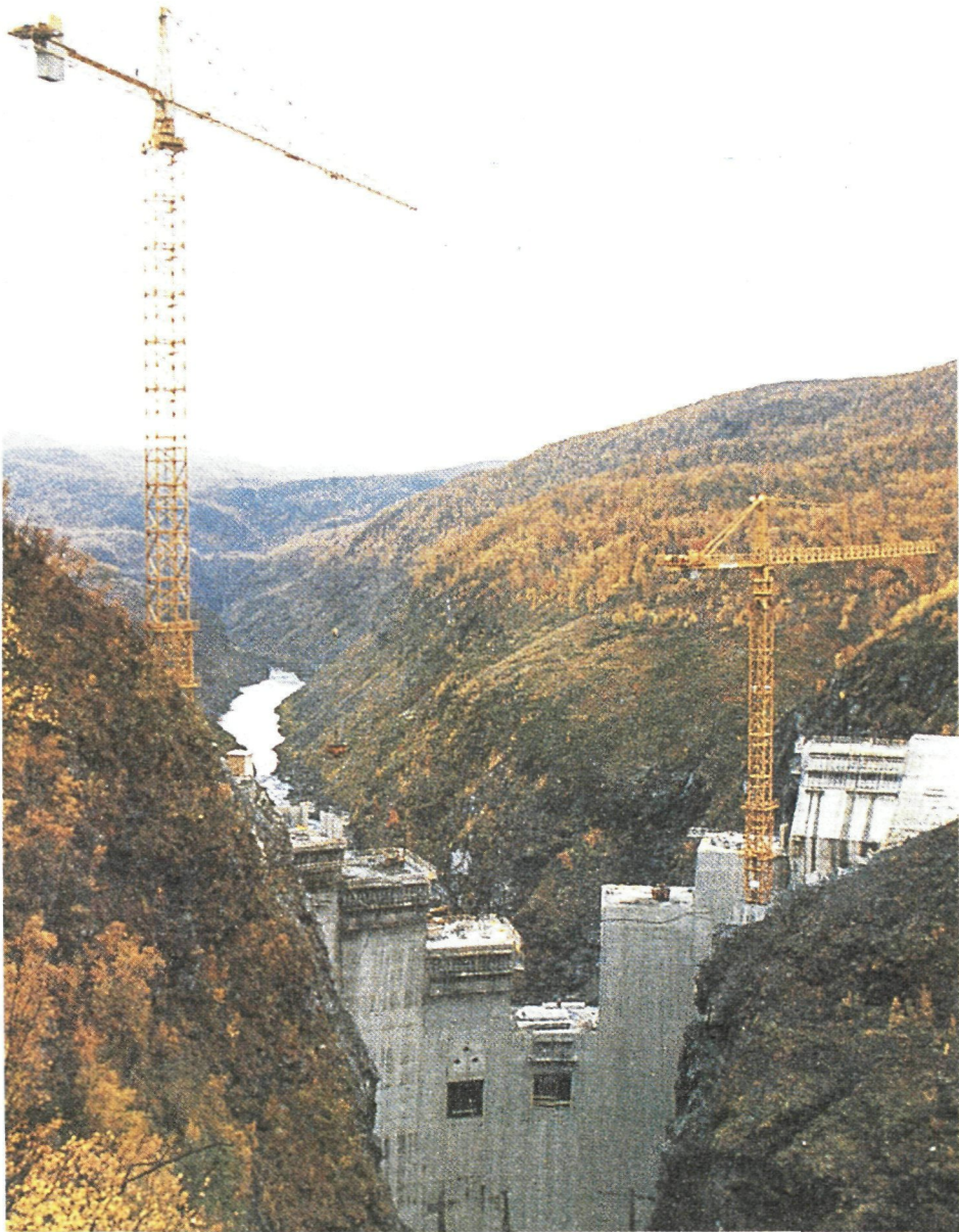
Fig. 1.3 The Virdejavre Arch Dam on the Alta River, under construction in 1987
