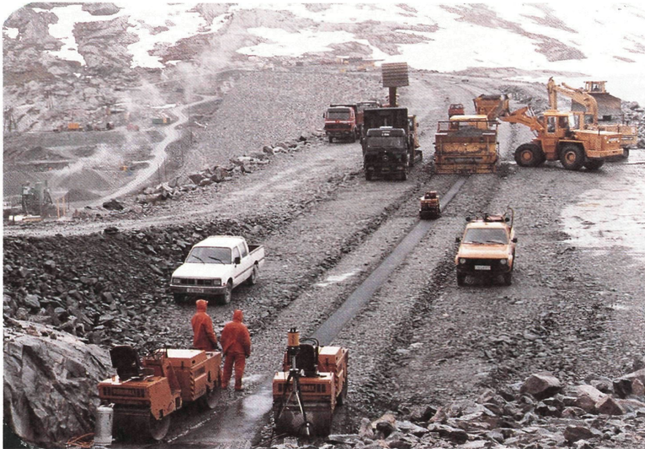
Fig. 4.1 The Norwegian asphaltic concrete paver at work on Styggevatn Dam
