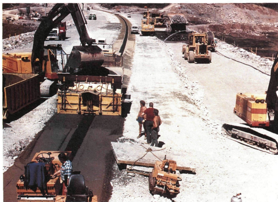
Fig. 2.1 Asphaltic concrete core construction for Riskallvatn Dam
