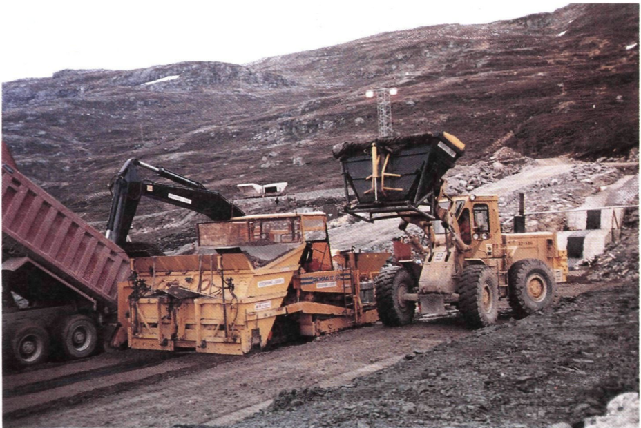
Fig. 4.5 Loading of asphalitic concrete and filter material into paver
