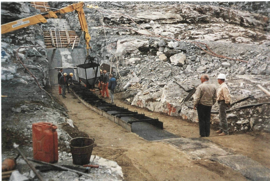
Fig. 4.6 Hand placement of asphaltic concrete
