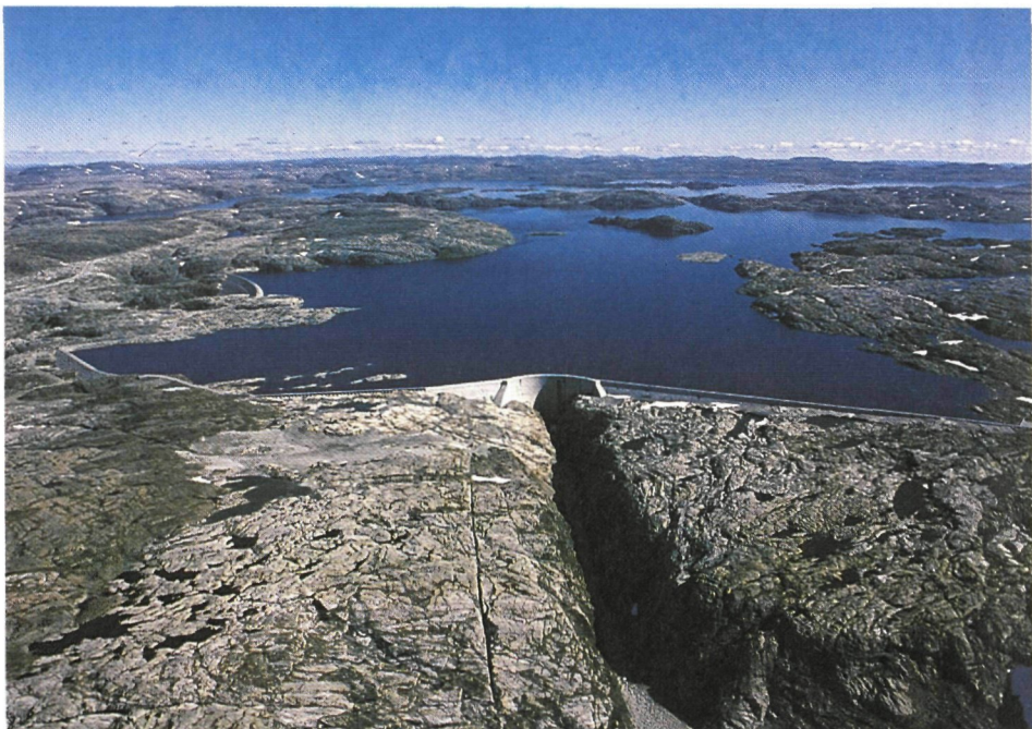
Fig. 1.1 The Blåsjø reservoir in mountainous West Norway
