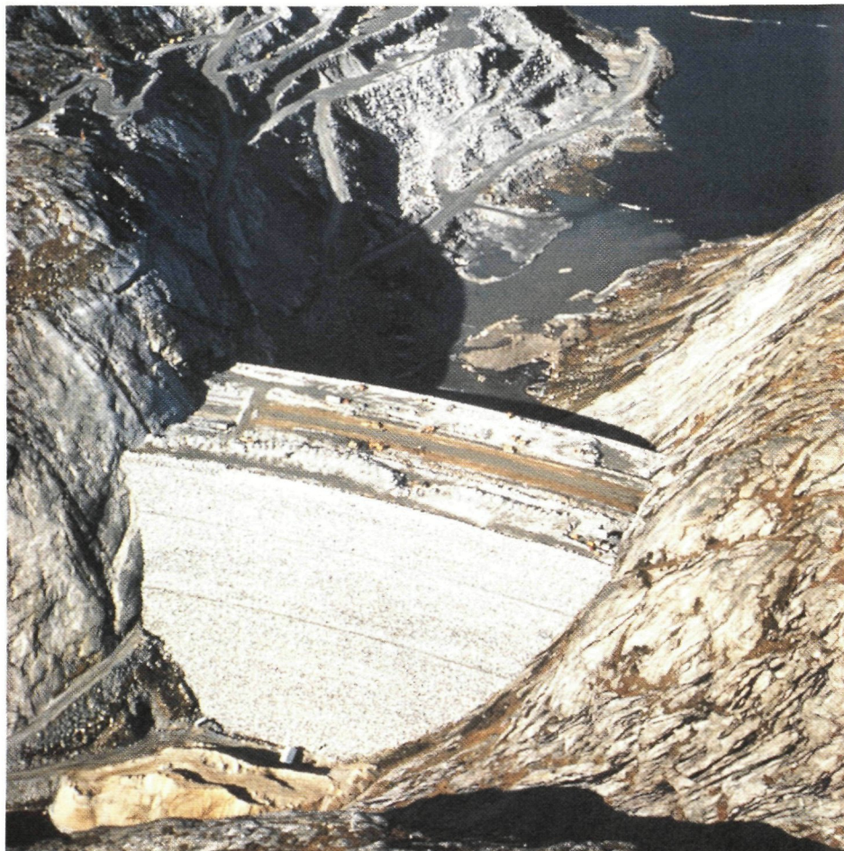
Fig. 1.2 The Svartevatn Dam (129 m high) with moraine core under construction
