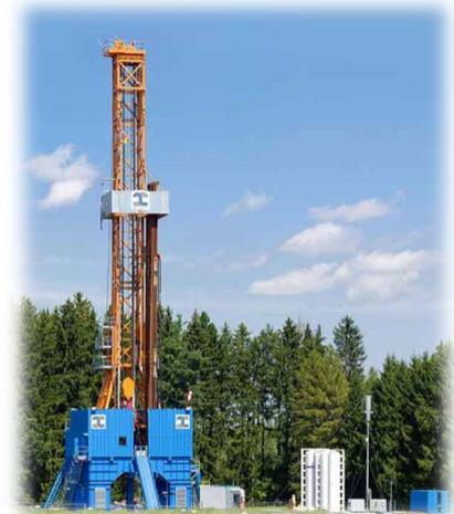
Figure 2.3 An image of a geothermal drilling rig during the construction. To reach the 70 C formation water at depth of 2.1 km, extensive drilling is required (Source: Energieoverheid, 2016).
