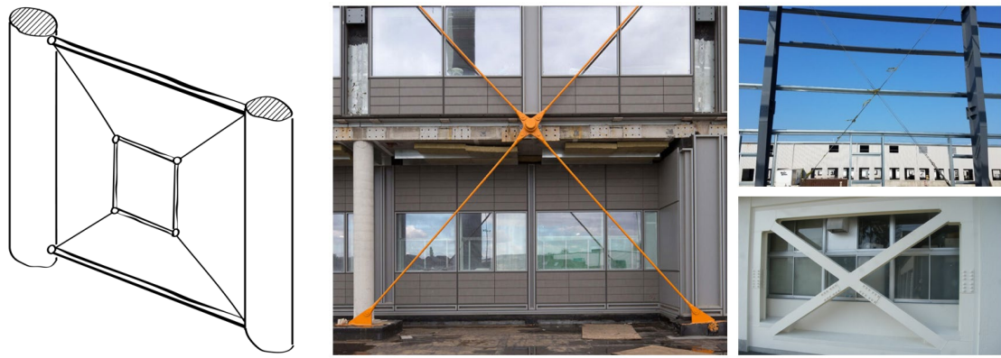
Figure 154: (4) Integration with structural cross-bracing. The system could benefit from larger structural elements, enabling higher cable pretensions. Buckling of the outer compression members would be less problematic.
