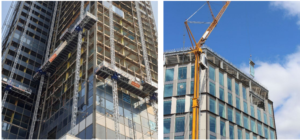
Figure 19: (left) mast climbing platforms and (right) tower crane installation (image sources: https://alimak.com/nl/product-category/mast-climbing-work-platforms/ & https://popsfacades.co.uk/unitised-curtain-wall-installation/ )
