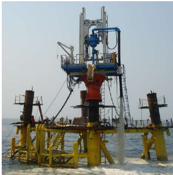
Figure 5.21: Example of a Wirth drill in operation on top of a pipe [1].
