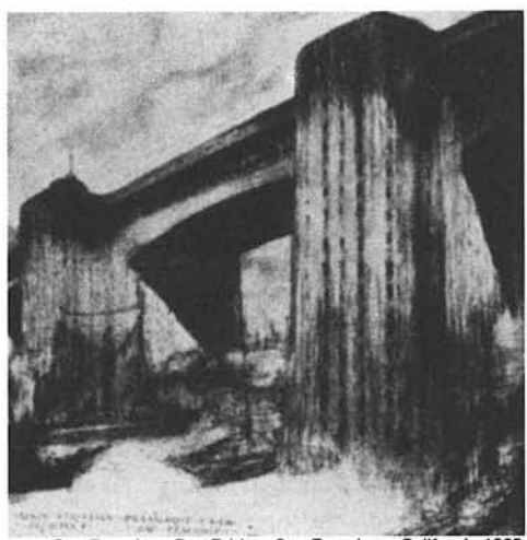
San Francisco Bay Bridge, San Francisco, California 1925
