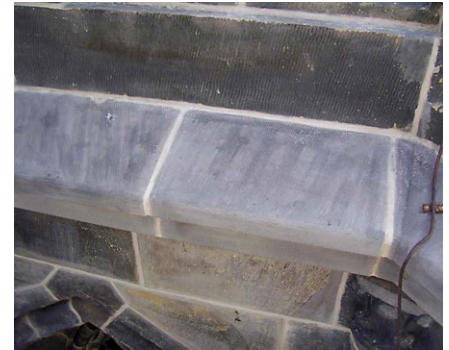
FIG. 2.14 Artificially patinated Bentheim sandstone on the lantern of the Laurens Church tower in Rotterdam / Photo: T.G. Nijland
