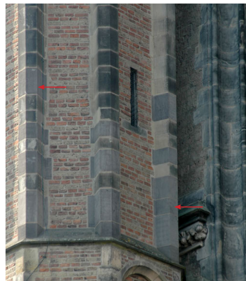
FIG. 2.9 Volvic basalt on the stair tower of the south transept of the Dom Church in Utrecht, as a replacement for Bentheim sandstone / Photo: W.J. Quist
