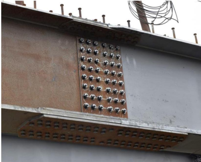
**Figure 1:** Double-lapped joint used for a splice connection [55]
