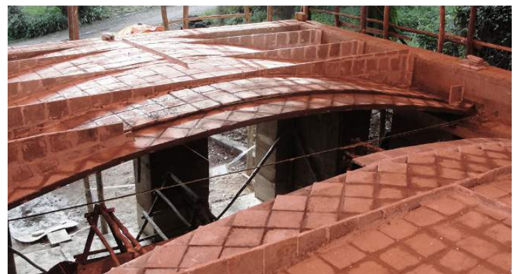
FIGURE 09: Catalan vault floor slab at SUDU project, Ethiopia with lightweight stiffening walls. Image retrieved from López López, D., Van Mele, T., & Block, P. (2016). Tile vaulting in the 21st century. Informes de La Construcción, 68(544), 162. https://doi.org/10.3989/ic.15.169.m15
