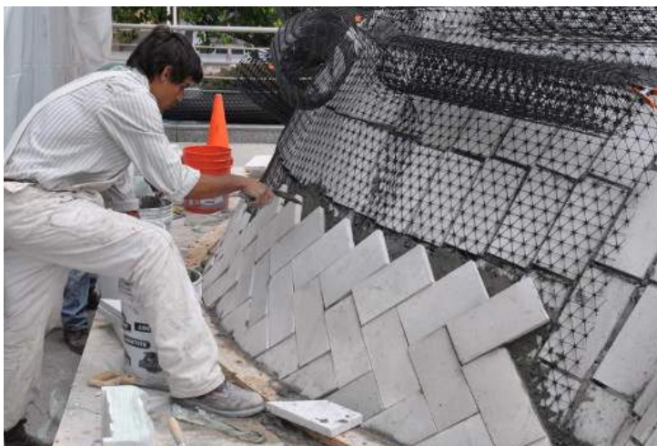
FIGURE 14: Geogrid embedded in between mortar layers and tiles, for reinforcement against seismic loads, in the Bows Centre, Yerba Buena Centre for the Arts, in San Francisco, USA. Image retrieved from Ramage, M. H., & Dejong, M. J. (n.d.). Design and Construction of Geogrid-reinforced Thin-shell Masonry.
