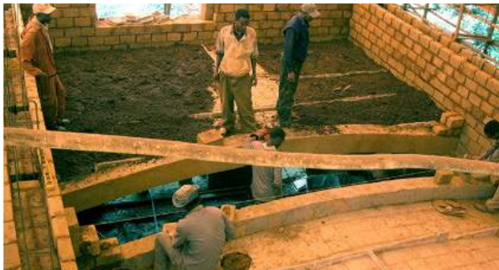
FIGURE 16: Catalan vault floor slab at SUDU project, Ethiopia, with lightweight stiffening walls and compacted fill. Image retrieved from López López, D., Van Mele, T., & Block, P. (2016). Tile vaulting in the 21st century. Informes de La Construcción , 68(544), 162. https://doi.org/10.3989/ic.15.169.m15
