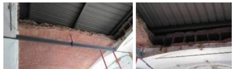
FIGURE 13: Partly demolished part of a Catalan slab showing vertical stiffeners in the hollow slab. Image retrieved from Nanayakkara, K. I. (2019). Shell Structures from Catalan to Mapungubwe Lessons from Structural Efficiency for Sustainable Construction in Developing Countries . https://doi.org/10.13140/RG.2.2.30878.89922
