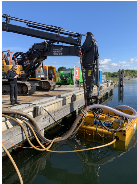
Figure 6.10: Testing at Werkhaven Bommenede
