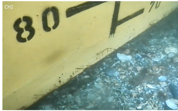
Figure 6.11: Photo of CDS on the bottom without turbidity with pump on
