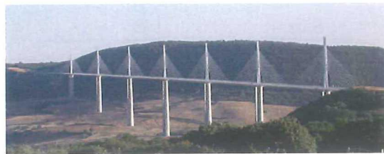
Fig. 7. Millau Viaduct bridge in France
