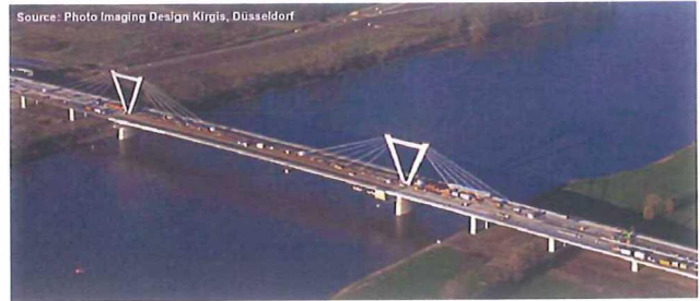
Fig. 6. Rhine bridge Dusseldorf-Ilverich
