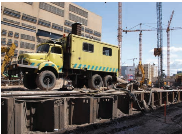
Figure 3 CPT truck during resistance measurements.
