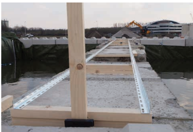
Figure 10 Top of test wall with track for positioning the potential electrodes.
