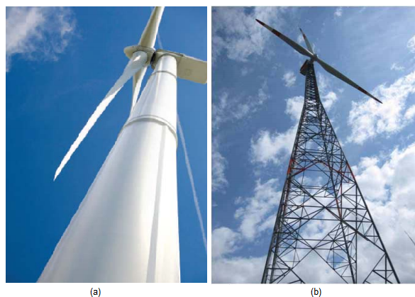
Figure 2.1: Common wind turbine tower designs (a) Tubular structure (b) Lattice structure [2]
