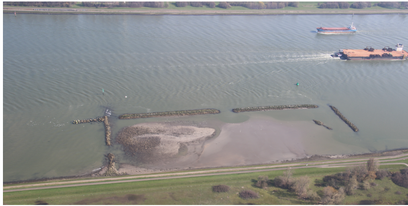
Figure 1.2: Aerial photo of Groyne Field 9 taken on 05-04-2023. The photo was taken at relatively low tide.
