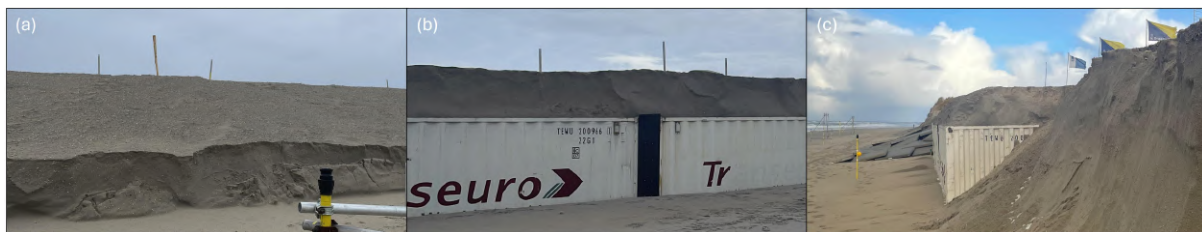
Figure 5.8: Overview of erosion progression in Section 4 (Wall-in-Dune). (a) 19-12-2024, 12:51 — Initial state before storm activity. (b) 23-12-2024, 14:28 — Erosion of the sandy layer and partial exposure of the container after Storm 2. (c) 02-01-2025, 14:39 — Continued downward erosion and stabilization of the dune face post-Storm 3.
