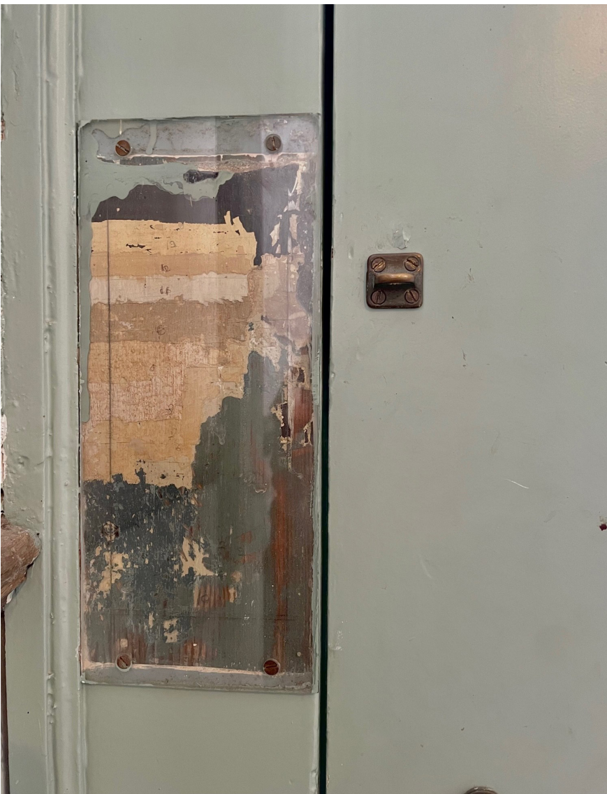
FIGURE 16. LAYERS OF PAINT ON THE FRONT DOOR OF OUDE DELFT 231. (OWN IMAGE)
