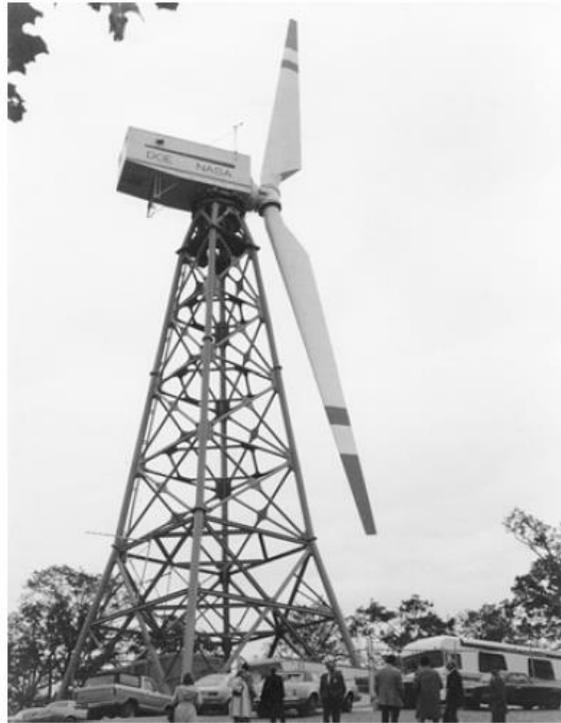
*Figure 3.2 MOD-1 (rotor diameter 61 m, 2000 kW, 1979 ) (Hau, 1998)*
