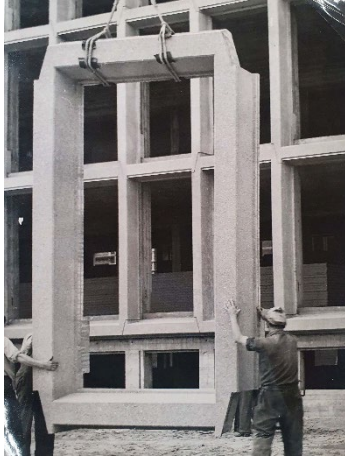
Figure 3. Mounting of the Schokbeton façade panels, The Hague municipal archives, 1958.
