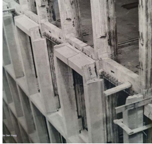
Figure 4. Connection of the Schokbeton façade to the concrete skeleton, The Hague municipal archives, 1958.
