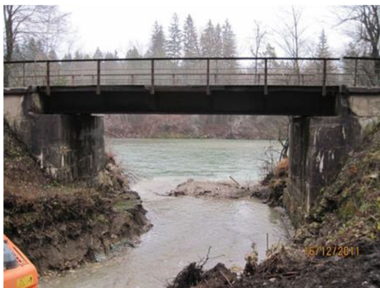
FIGURE 8 Scour of foundation at Plaznica bridge on the line between Ljubljana and Jesenice (Gavin, 2016)
