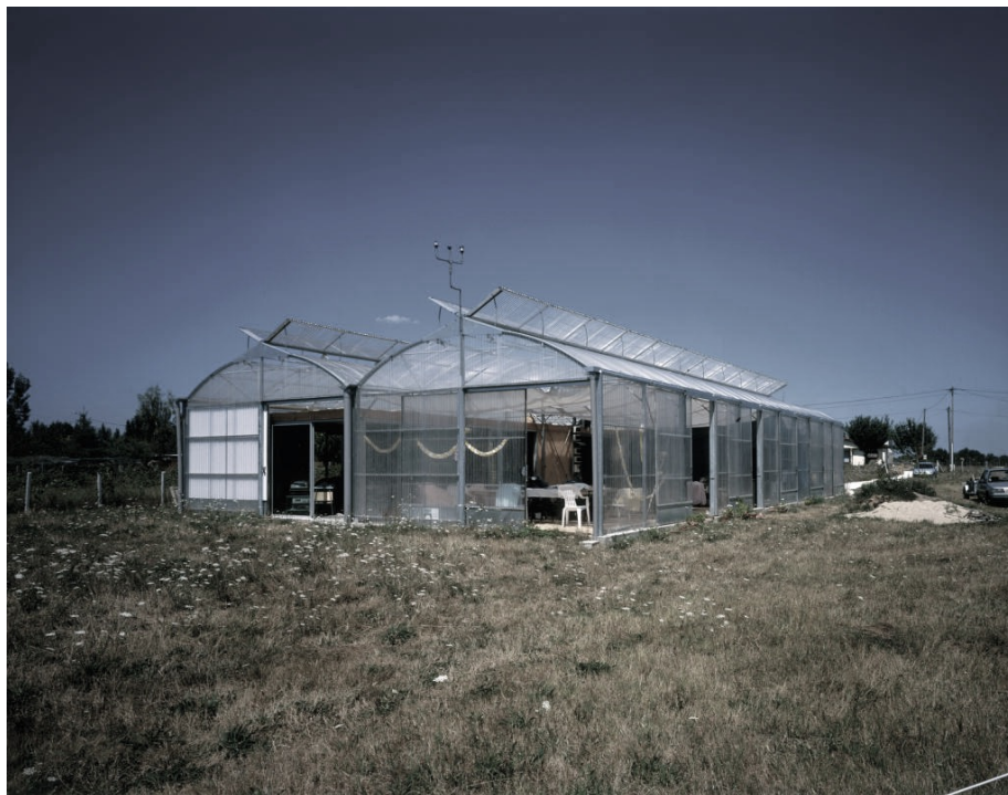
Image 9. House in Coutras (2000), by Lacaton & Vassal
