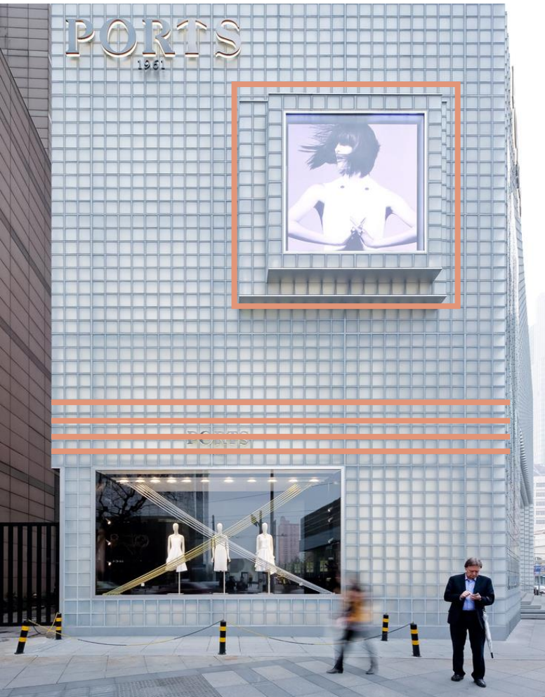
Existing building façade – hollow block
