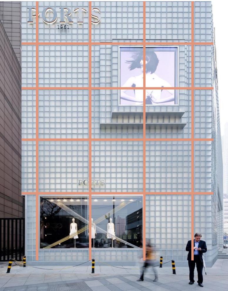
Existing building façade – hollow block
