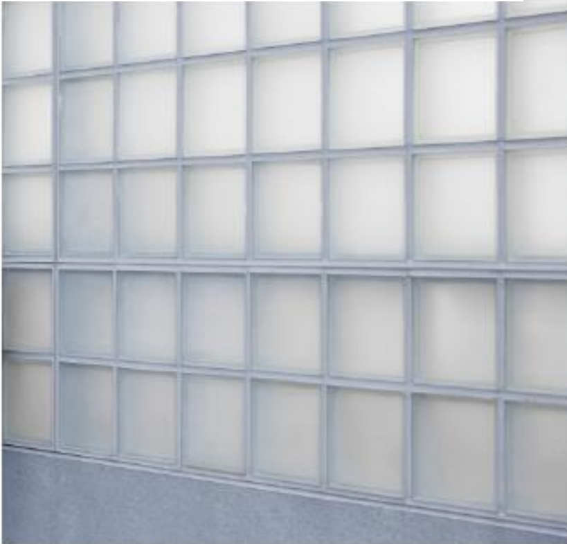
Existing building façade – hollow block
