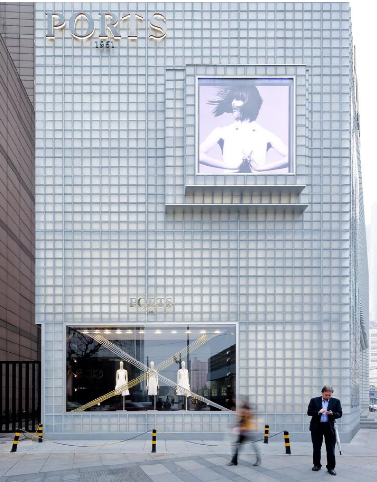
Existing building façade – hollow block
