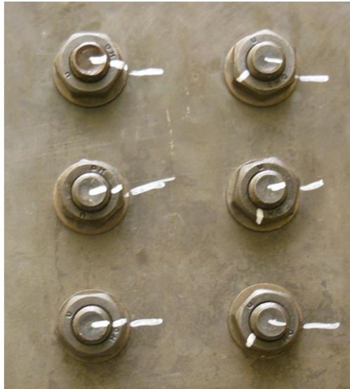
**Figure 2-5:** Marking of bolted connections to determine whether the bolts have turned during operation (source: [www.appliedbolting.com](http://www.appliedbolting.com))
