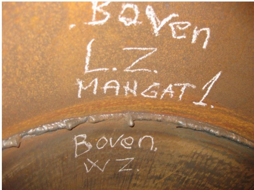
**Figure 3-2:** A weld applied from the outside of the connection, as pictured from the inside of the structure (image provided by Cargotec).
