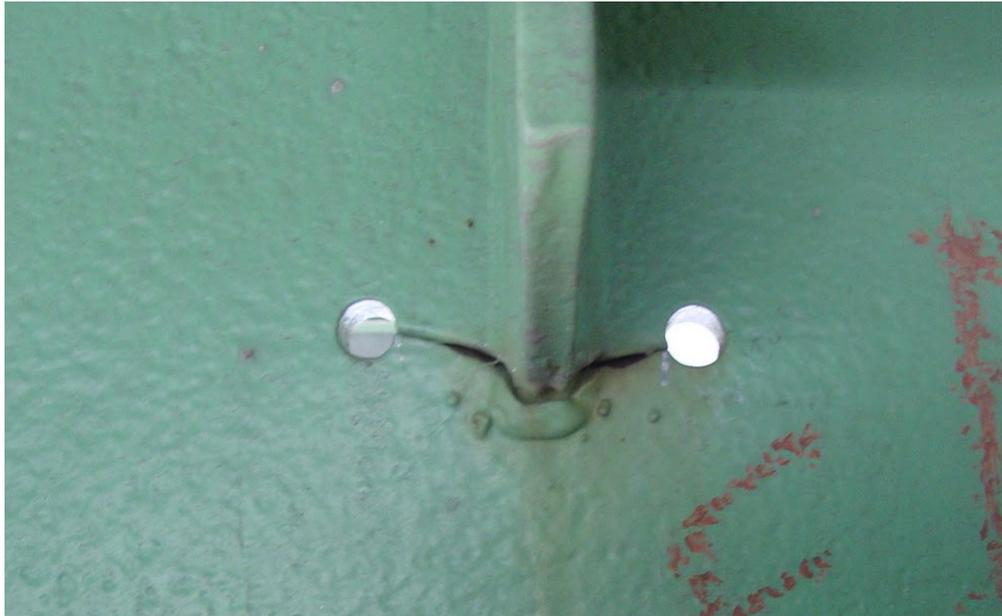
**Figure 7-4:** Two crack arrest holes are used to stop a center crack which is initiated at a welded detail (source: [www.alwayscivil.blogspot.com](http://www.alwayscivil.blogspot.com)).
