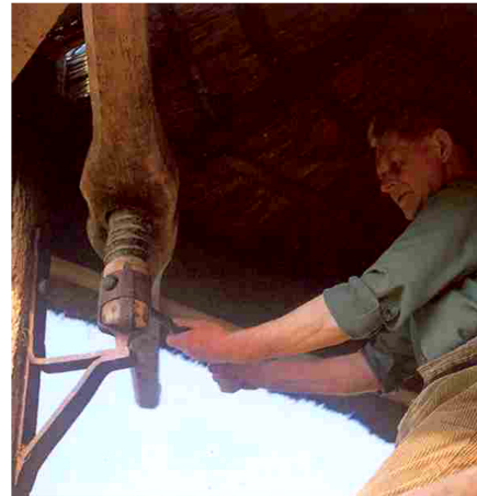
Figure 7.16: A screw or 'ronsel' worked as a conventional jack. Image from: www.hooiberg.info [19].
