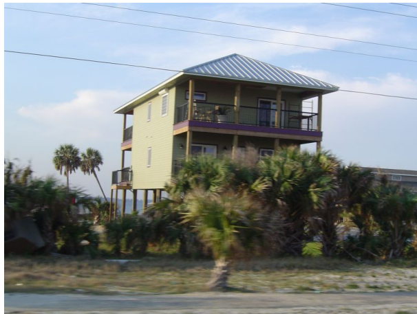
Figure 7.4: Pier column foundation in Gentilly District, New Orleans.
