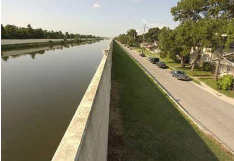
Figure 5.6: Floodwall in New Orleans. Image from: NOLA [23].
