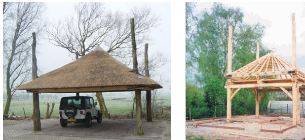
Figure 7.13: Hay barrack in use and during construction. Image from: www.hooiberg.info [19].
