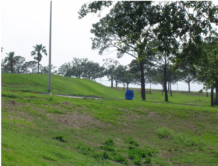
Figure 5.1: The present peripheral levee (picture taken on top of the berm).
