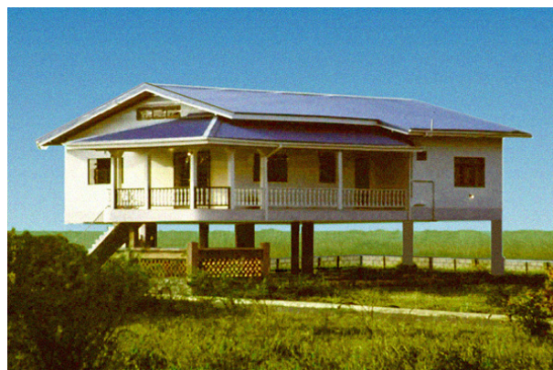
Figure 7.6: Pile house in Florida.
