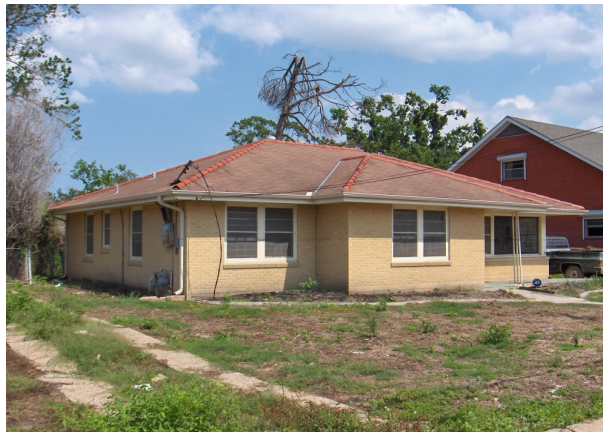
Figure 7.2: Slab-on-grade building in Gentilly District, New Orleans.
