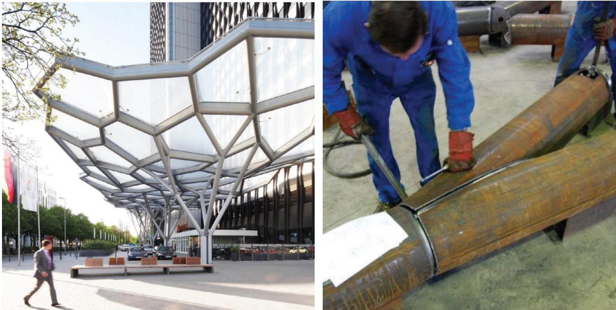
Figure 1.1: The Westend Gate Tower canopy [5]. Left: Structure overview. Right: The assembly and welding of grid shell canopy compartments.
