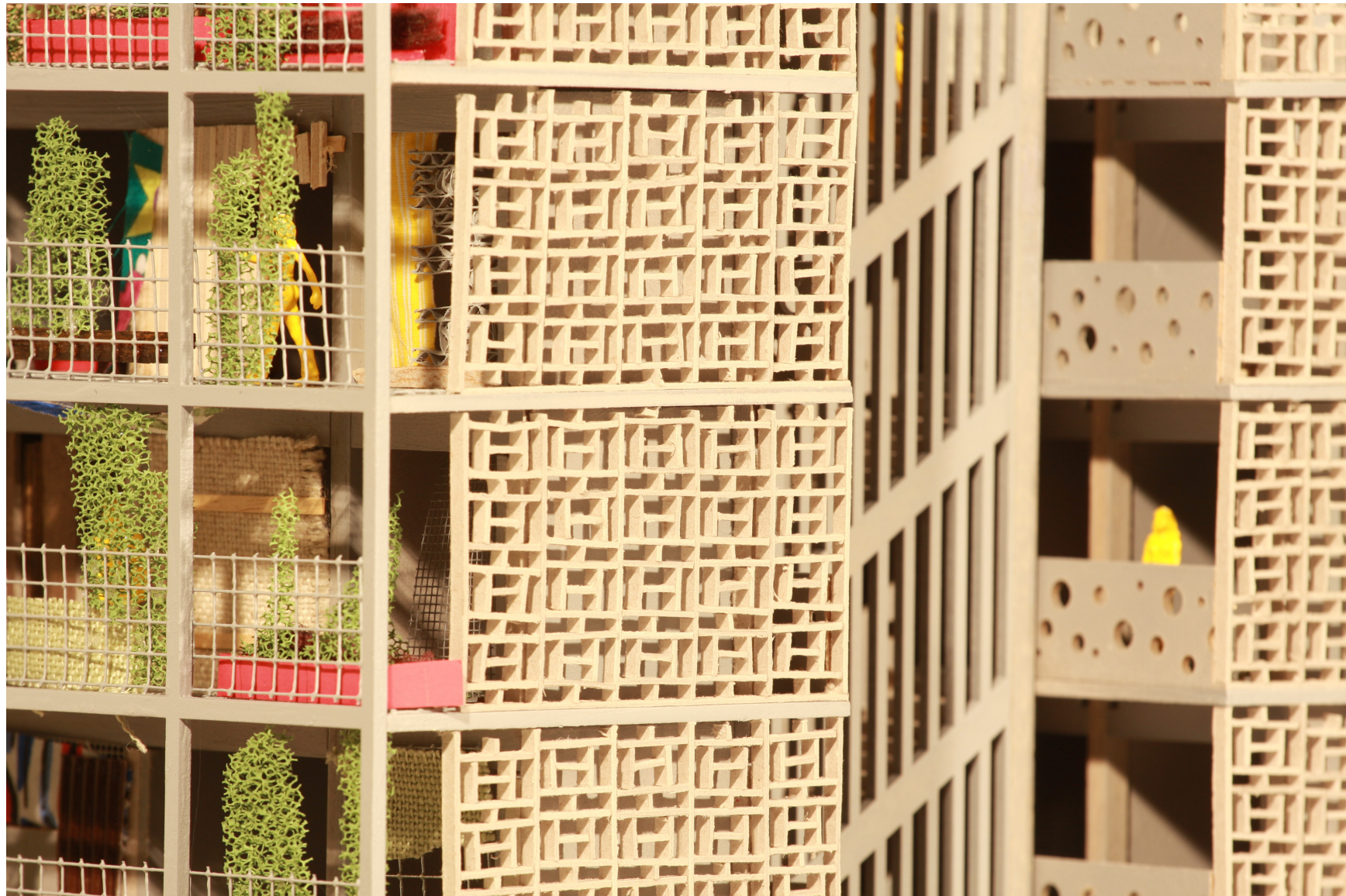
Figure 3.24: the texture on the northwestern facades creates a characteristic image, relating to the frivolous textures seen elsewhere in Maputo, but also stands in contrast with the informal and less structured other two facades of the building, which are to be "coloured in" by the inhabitants.
