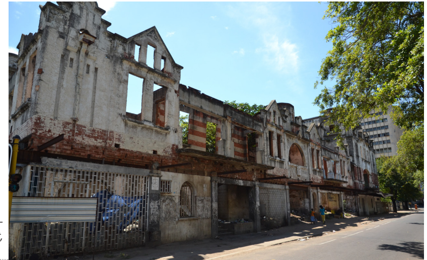
Figure 4.12: long facade of Predio Pott, on a Sunday. (MvB)
