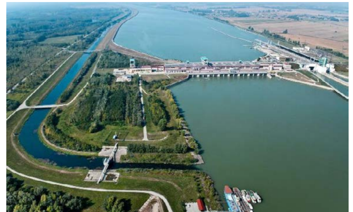
Gabcikovo Dam (Google.com, 2014)
