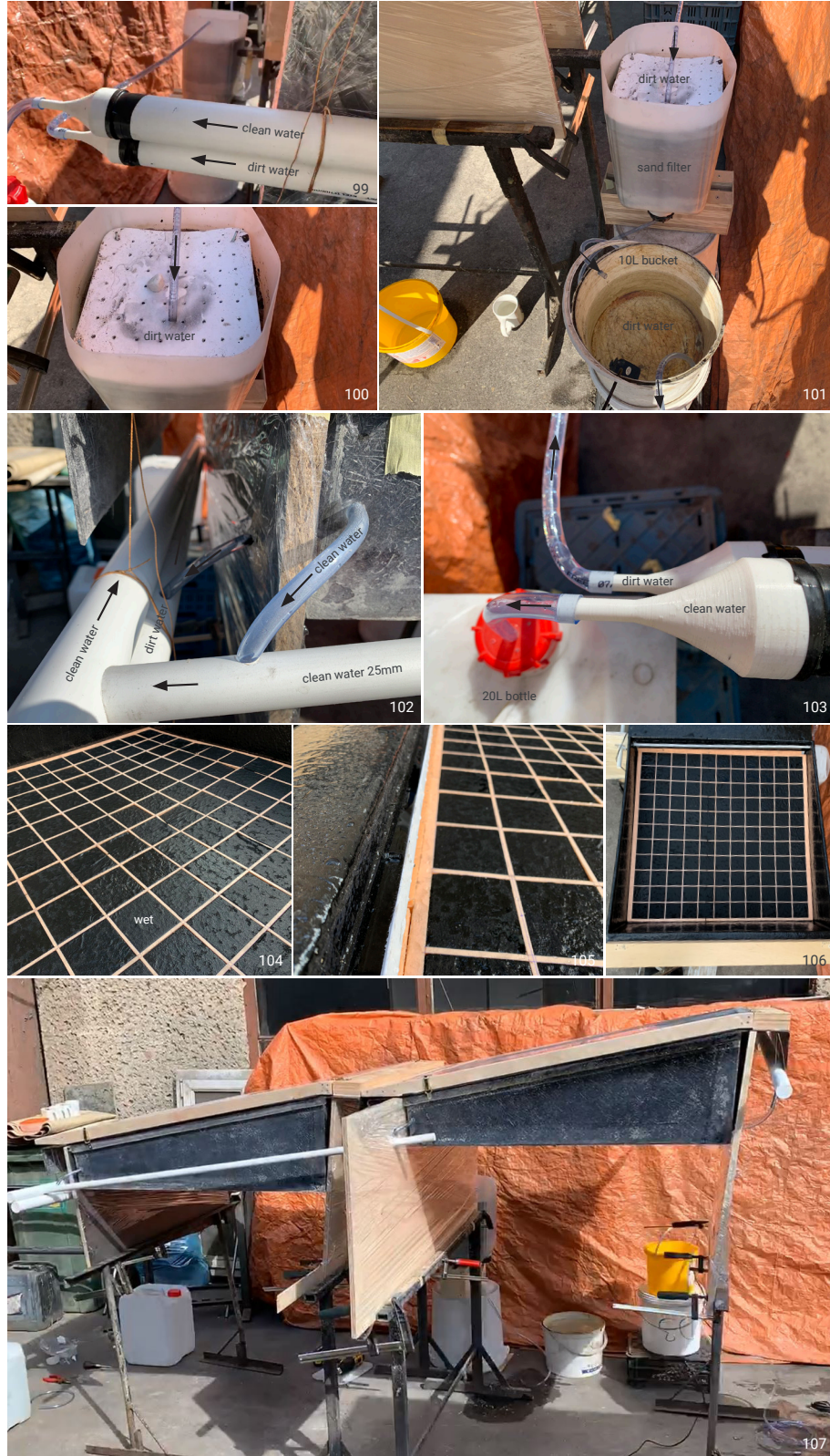
Phot. 99-107 Mock-up assembly steps. Author's photography.
