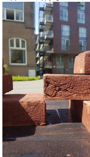
(e) T=16:22, failure with two bricks;
