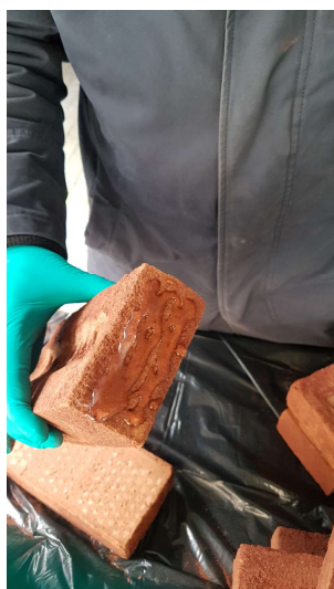
(a) T=15:35:11, applying adhesive;
