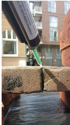
(b) T=1:03, applying additional adhesive;
