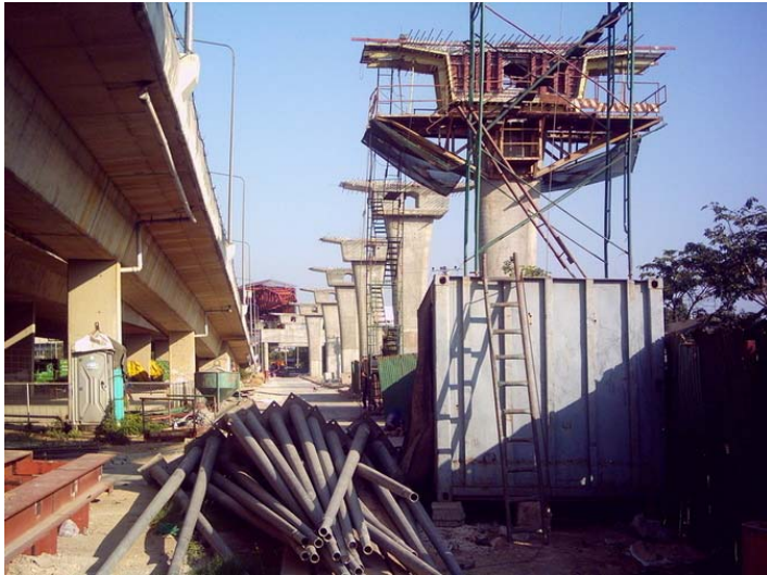
Figure 19: Cast in-situ columns with box girder segment
