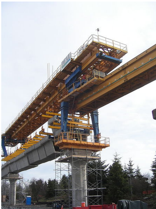
Figure 10: Construction of the girders using a launching truss
