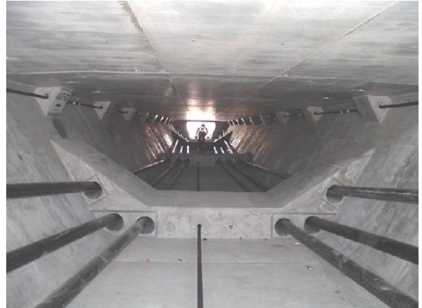
Figure 7: External prestressing tendons in the box girders
