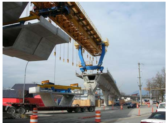
Figure 9: Construction of the box girders using a launching truss
