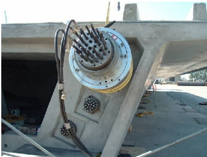
Figure 8: Post-tensioning of a bundle with strands
