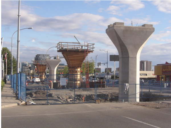
Figure 6: The columns cast-in-situ
