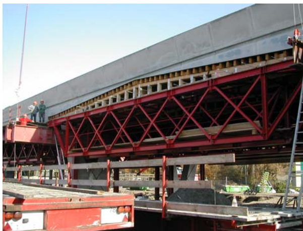
Figure 26: The tapered railway structure supported by a falsework
