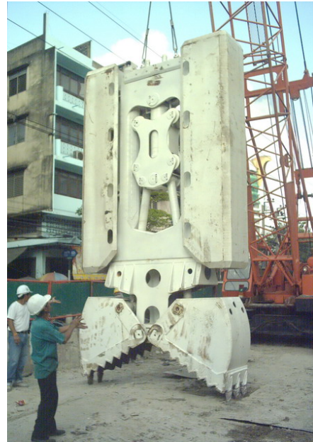
Figure 20: Excavation using a grab for the construction of a barrette pile
