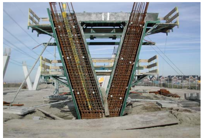
Figure 27: Reinforcement of the V-columns
