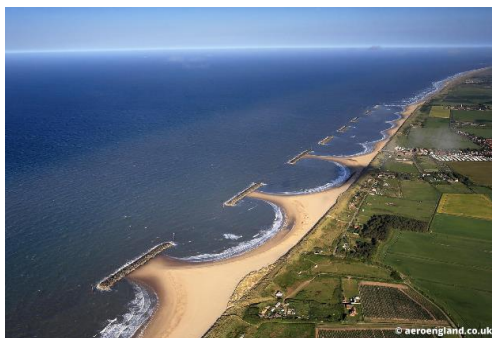
Figure L1: Breakwater at Sea Palling, Norfolk UK. (J. Webb, 2015)
