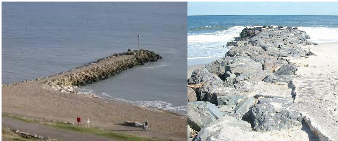
Figure L11: Rubble-mound breakwaters L: Stacey, A. (2011) [Photograph]. Retrieved from http://www.stacey.peak-media.co.uk/Highcliffe/800-10210015.jpg R: Unknown. (n.d.) [Photograph]. Retrieved from http://wikivisually.com/wiki/File:Sea_Bright_Beach_Jetty.jpg
