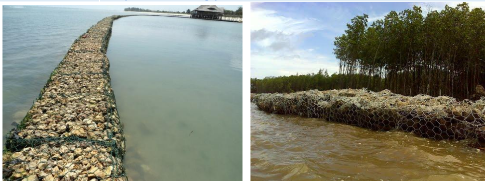
Figure L10: Gabions (Bá Lọc. (2013, September 28). [Photograph]. Retrieved from Google Earth)
