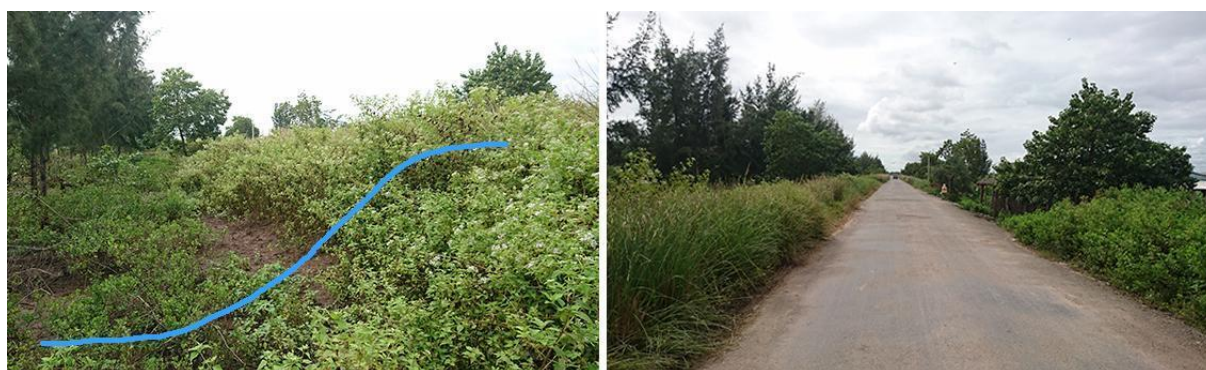
Figure 7: (l) Side view sea dyke; (r) Crest including road of the sea dyke at Bạc Liêu
