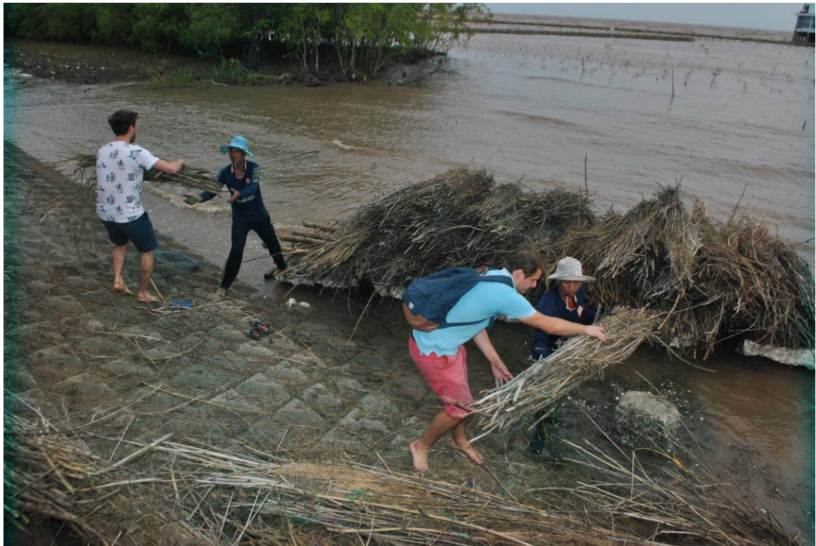
Figure E2: Preparations to refill the fences
