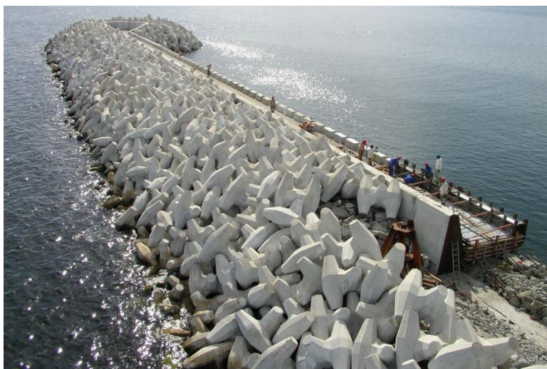
Figure L2: Breakwater at Fujairah (A.d. Grauw, n.d.)
