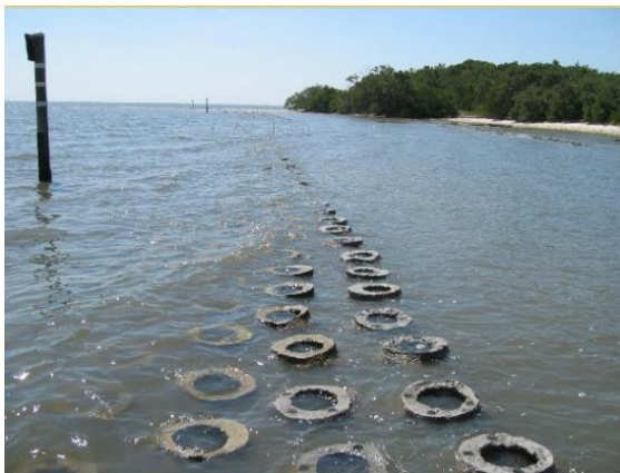
Figure L5: L: Reef balls to create oyster bars for shoreline stabilization (Unknown. (n.d.). [Photograph]. Retrieved from http://www.reefbeach.com )
