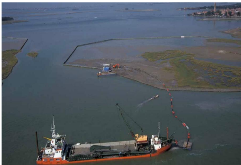
Figure L15: Direct nourishment (Cecconi, G. (2009) Beneficial Reuse and Morphological Restoration , SedNet Conference 2009, Hamburg, Germany)
