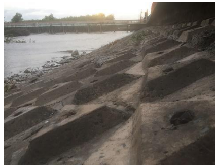
Figure 19: Dyke revetment at Nhà Mat Community
