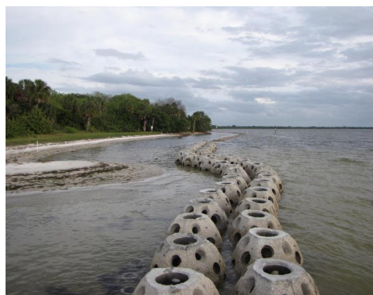
Figure L6: Oyster reef breakwater (FCIS staff. (n.d.). [Photograph]. Retrieved from http://fl.audubon.org/news/oyster-reef-breakwater-lengthened-protect-major-tampa-bay-nesting-rookery )
