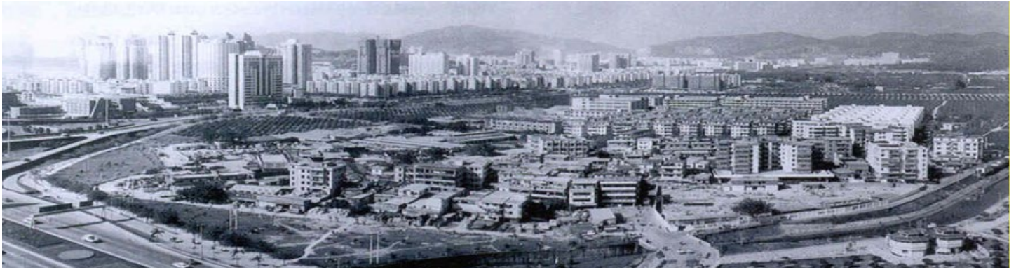
Figure1.1.2.1 Tianmian village in 1990s
