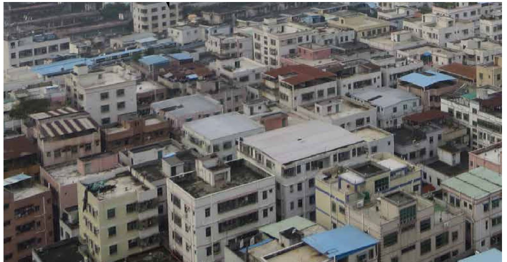
Figure 6.2.1.7 The image of roof in Baishizhou Source: http://sz.southcn.com/s/2014-09/05/content_108011434.htm
