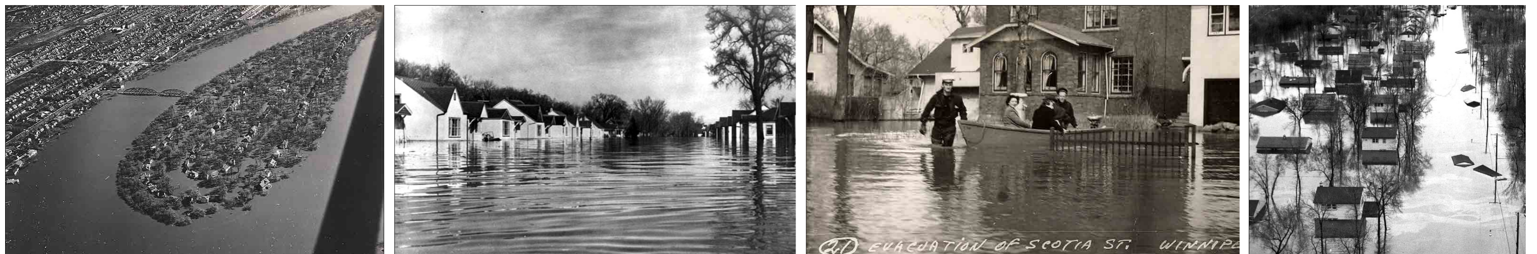
Figure 1-3: Photos of the devastating flood that washed over Winnipeg Source: City of Winnipeg, 1950
