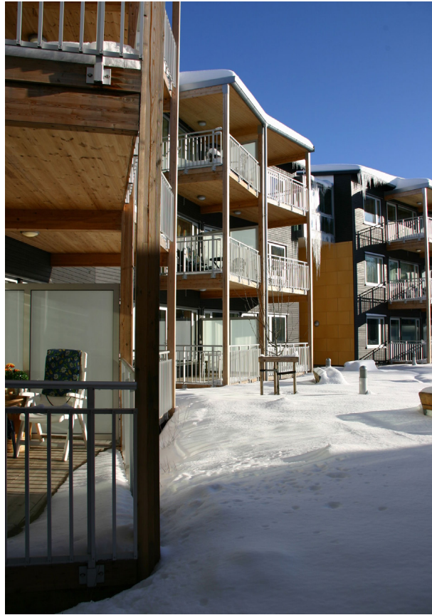
Figure 5.2.14 | Picture of Tarnasen Housing and Activity centre (Fedderson & Ludtke, 2018)
