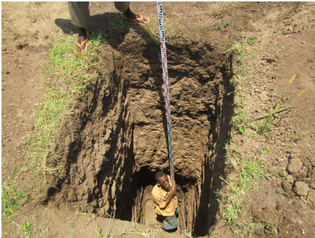
Figure 13. Trench excavation inside Roseires Reservoir.
