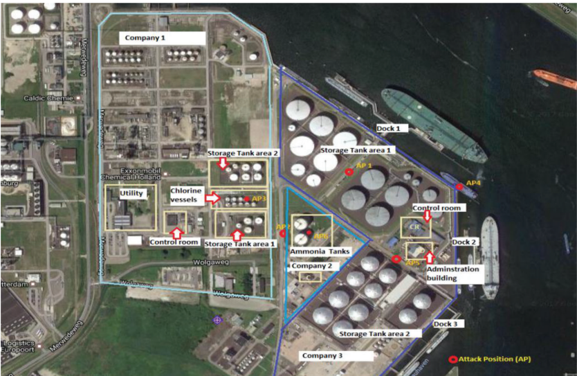
Figure 4: Chemical cluster comprising three chemical plants.
