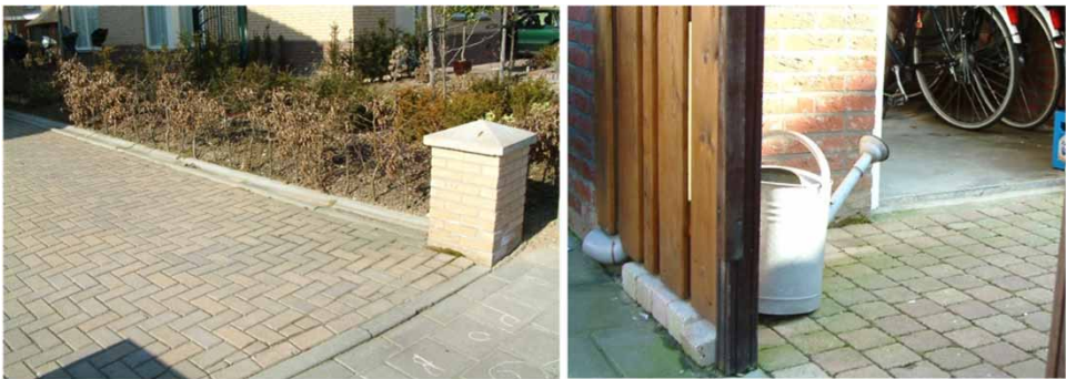
Figure 1 | Two cases (#13 and #15) of technical failures in SUDS with a failing function of conveyance. Left: an obstacle interferes with the transport of water by an open gutter. Right: due to insufficient slope of the garden, the storm water flows into the shed.
