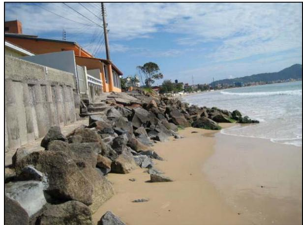
**Figure E-2 Property protected by dump stones and seawall. Northern headland in background.**
