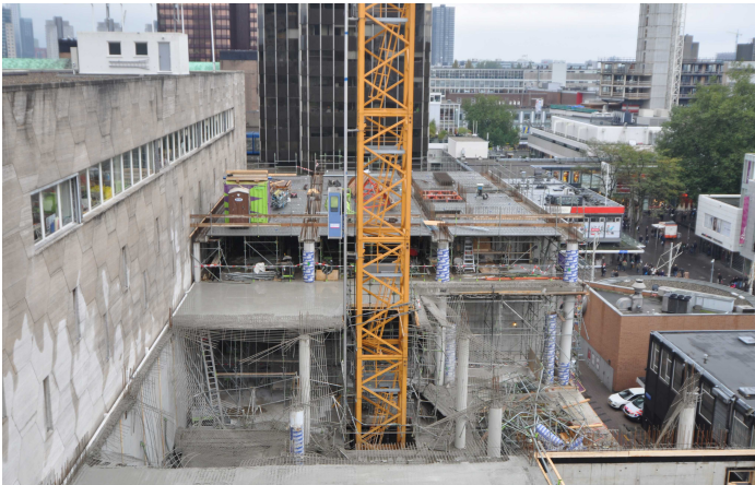
Figure 7.2 Top view of collapsed floor B-tower (photo: Karel Terwel)
