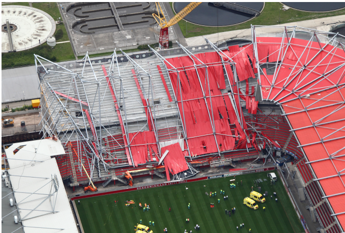
Figure 7.3. Roof of FC Twente stadium after collapse. Reproduced by permission of the Netherlands Police Agency, Air support and Aviation Police
