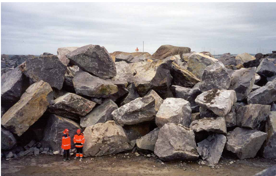
Figure 1.2 Sirevåg berm breakwater, stock pile of stone classes I and II. Sigurdarson et al 2001
