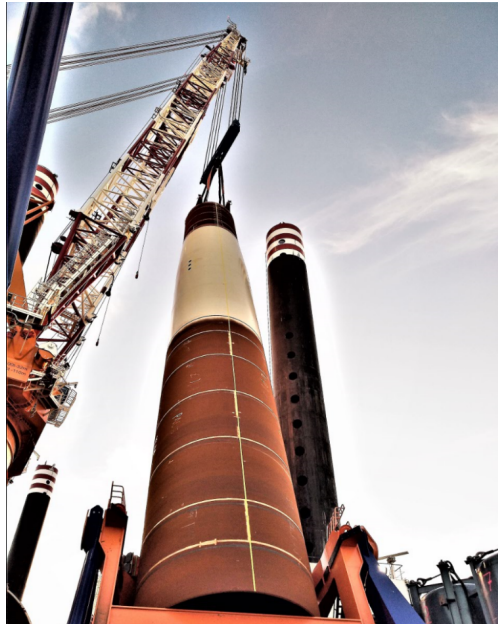
Figure 2.7: Uniform corrosion on a monopile at the Aeolus
