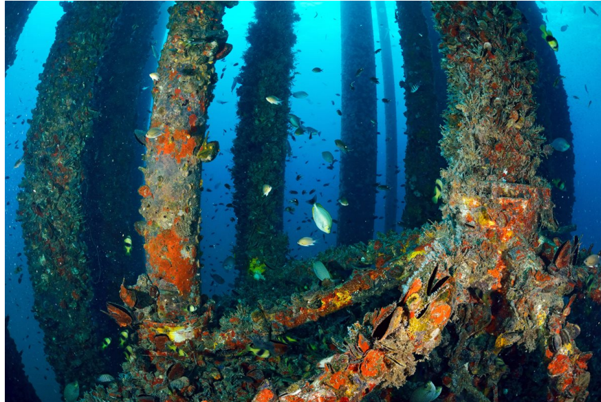
Figure 2.6: Example of biofouling in marine environment [12]
